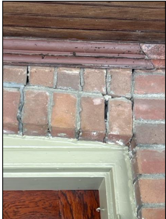
Mortar deterioration
