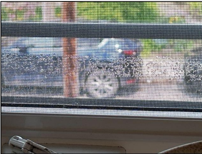
Lost seal on double or triple glazing
