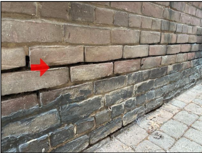
Mortar deterioration
