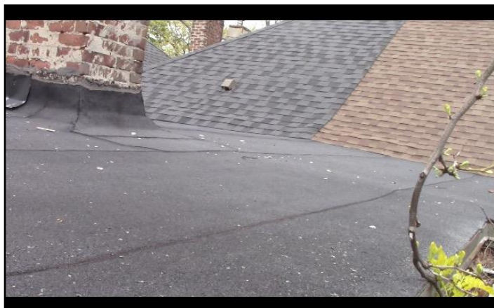
Modified bitumen membrane
