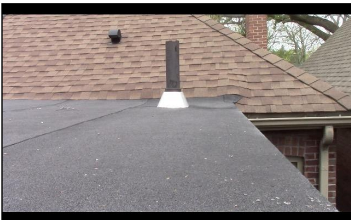
Modified bitumen membrane
