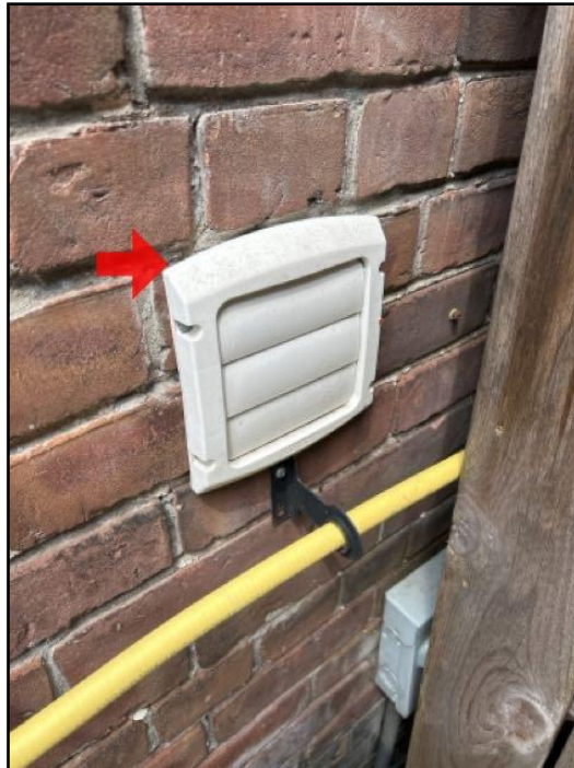
Caulking deteriorated/missing
